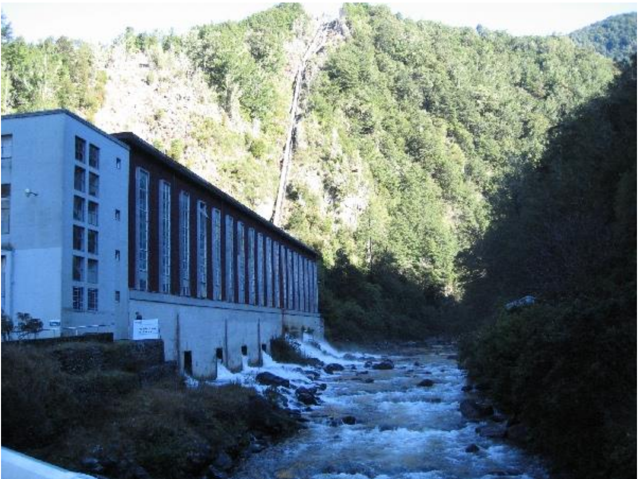
Figure 3-7: Cobb Power Station (taken from trustpower.co.nz ).
